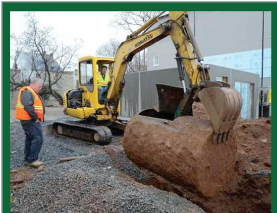
**STEVE RICH & ASSOCIATES ENVIRONMENTAL CONTRACTORS**, removes a 500-gallon underground oil tank at a Paterson site for Habitat for Humanity; Rich, at left, prepares to examine the tank. Below left, worker Justin O'Connell uses a dipstick to check a second tank on the site for the presence of water.
